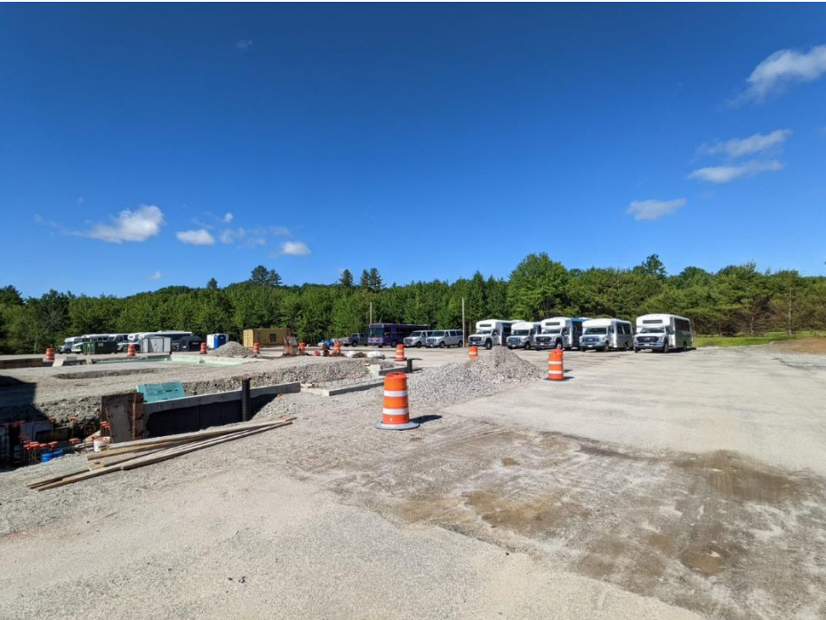
Figure 7 WMTS Facility Parking Area and New Maintenance Bays Under Construction
